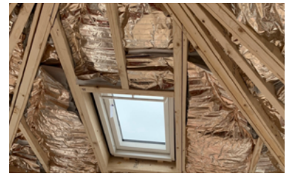
Internal roof insulation pre plastering.
